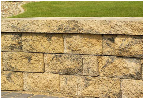
Split-face concrete block wall with cap
