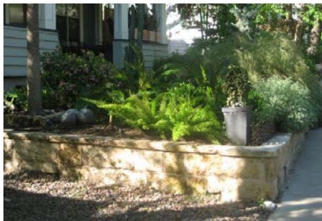
Masonry wall with cap
