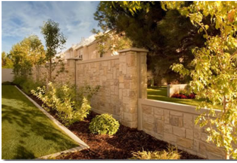
Six foot high privacy masonry wall
