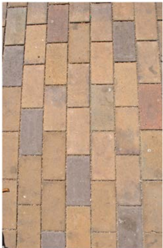
Concrete Permeable Pavers (Eco-CityLock by Pavestone, or Aqua Rock by Old Castle), “Mueller Blend”, Running Bond Pattern
