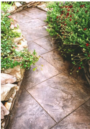
Stamped & stained concrete
